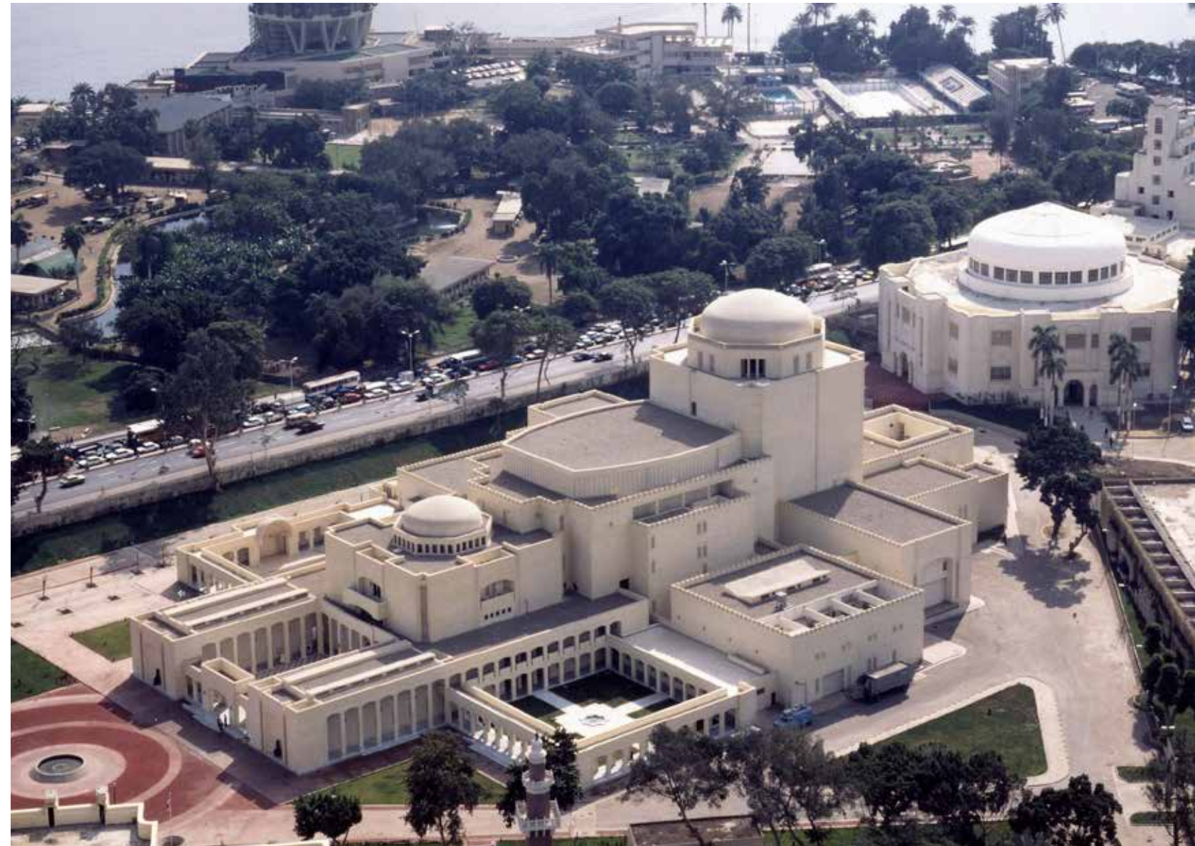
Overall bird's-eye view at the time of completion
