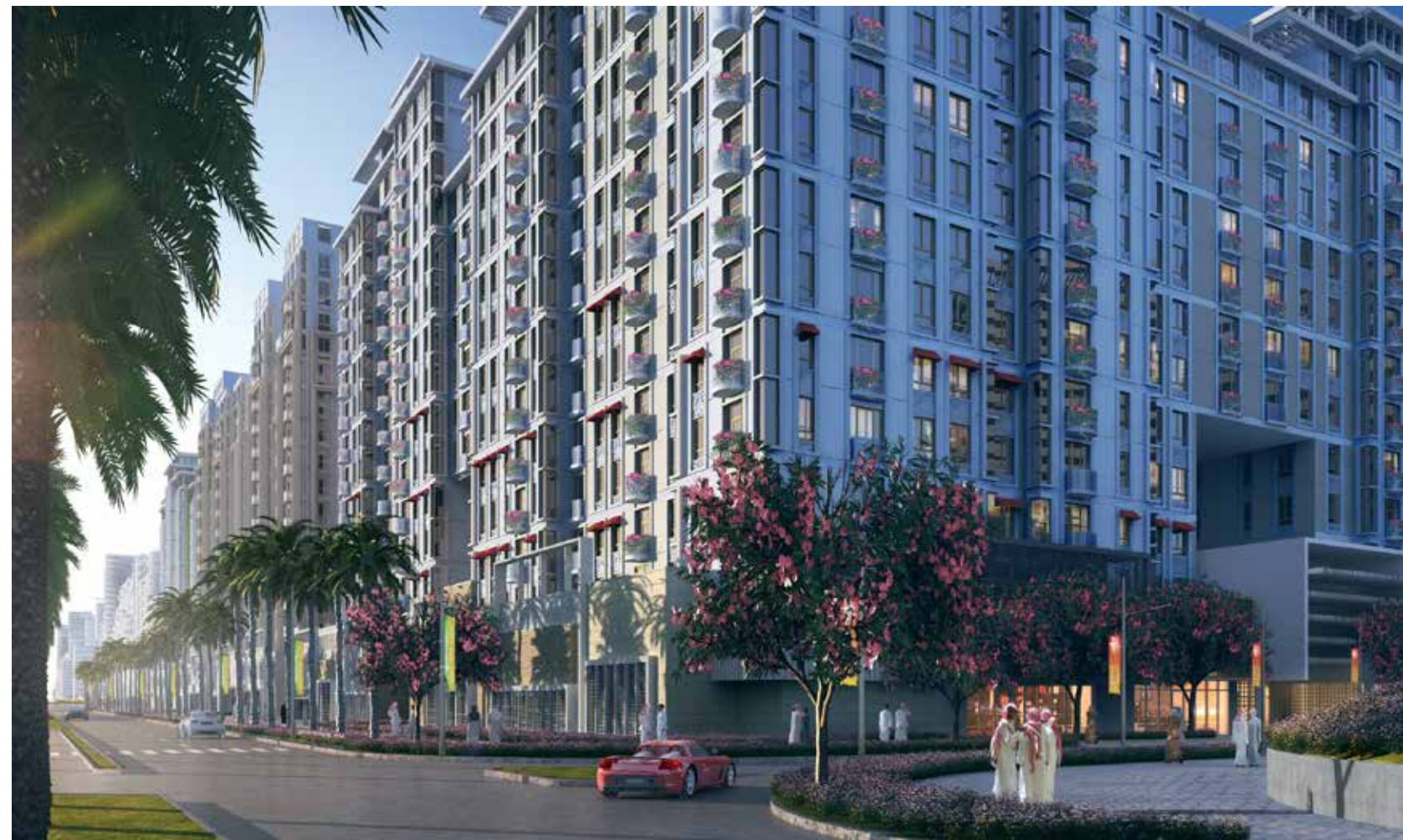
Approach towards the first residential block (currently under construction)
