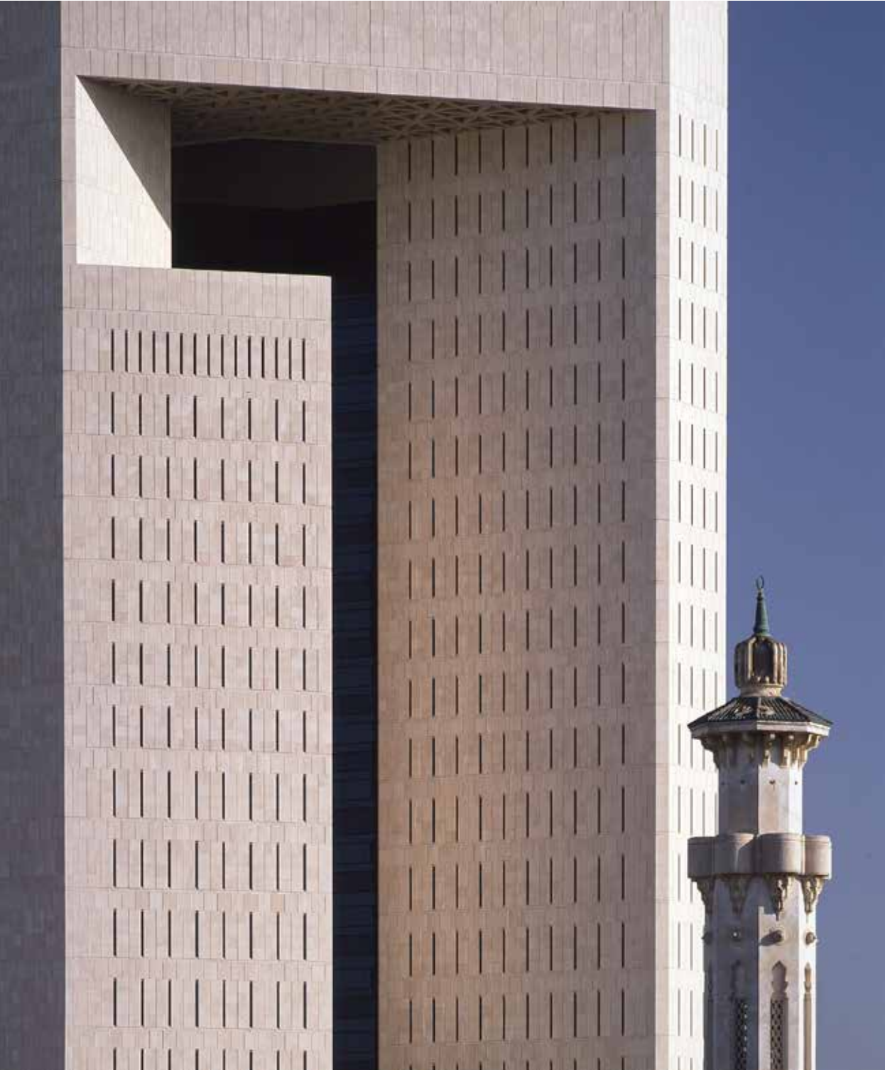
Close-up of the façade, the stone-clad exterior sheltering and shading the curtain wall
