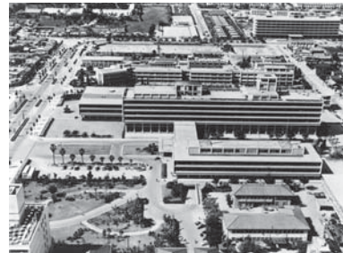
3-14 Hiroshima New Prefectural Office (1956).
