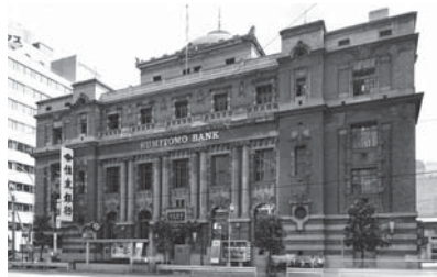
2-1 Sumitomo Bank, Tokyo Branch Office, 1917.
